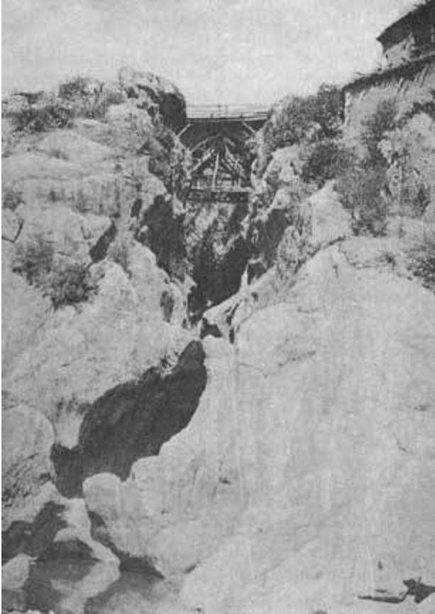
Bridge at Zeitun
